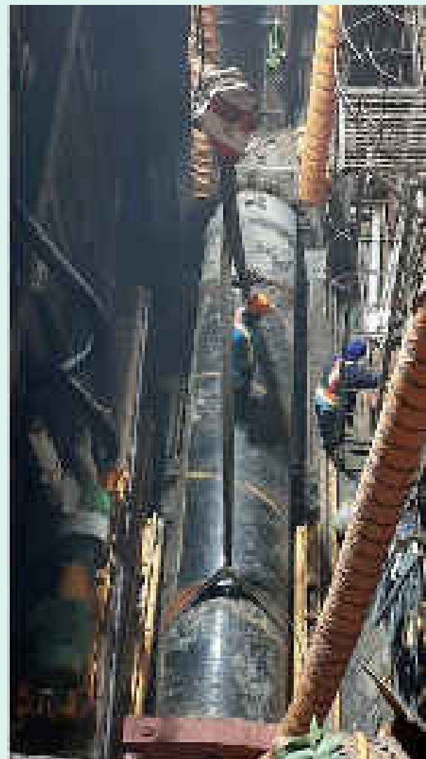
Construction of the SLEX Pipe Crossing Project
